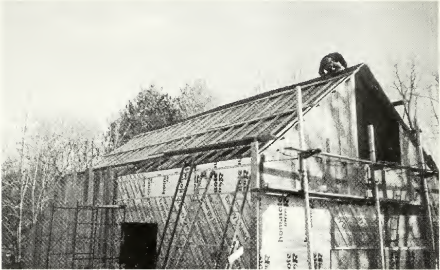
The barn before the roof was completed and the exterior vertical siding was applied
